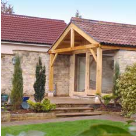
Finished sun room
