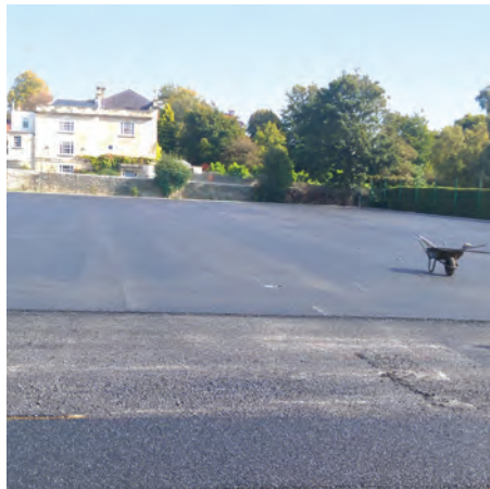
Laying porous sports macadam
