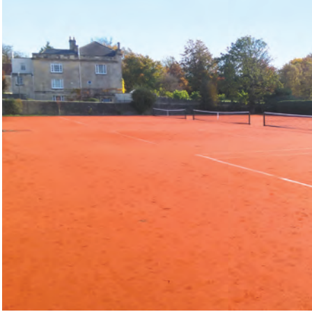
Completed red courts
